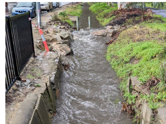
Existing degraded drainage channel during rainfall event which presents a public safety hazard
